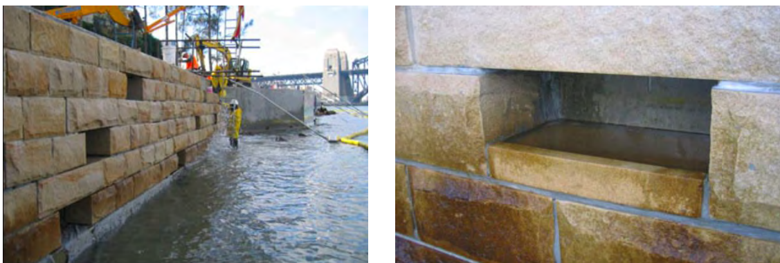
Fig. 2.8: Intertidal ‘rock-pools’ built into the vertical face of a sea wall in Sydney Harbour Australia, designed to retain water during low tide. Reproduced from Bulleri and Chapman (2010).
