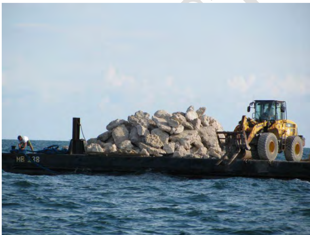
Fig. 2.1: Dumping of quarry rock and concrete rubble for the creation of an offshore artificial reef. Reproduced from Nell (2010).
