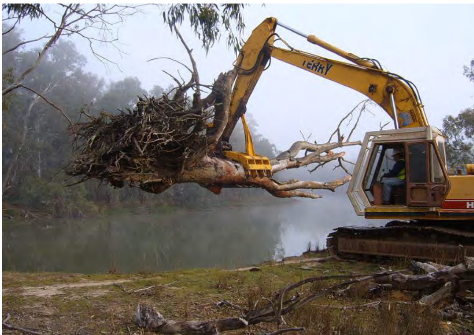
Figure 18: Large snag being installed on the Murray River (Source: Fish Habitat Network).
