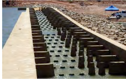
Above Glenore Weir Cone Fishway (high flow) located in the Southern Gulf of Carpentaria
