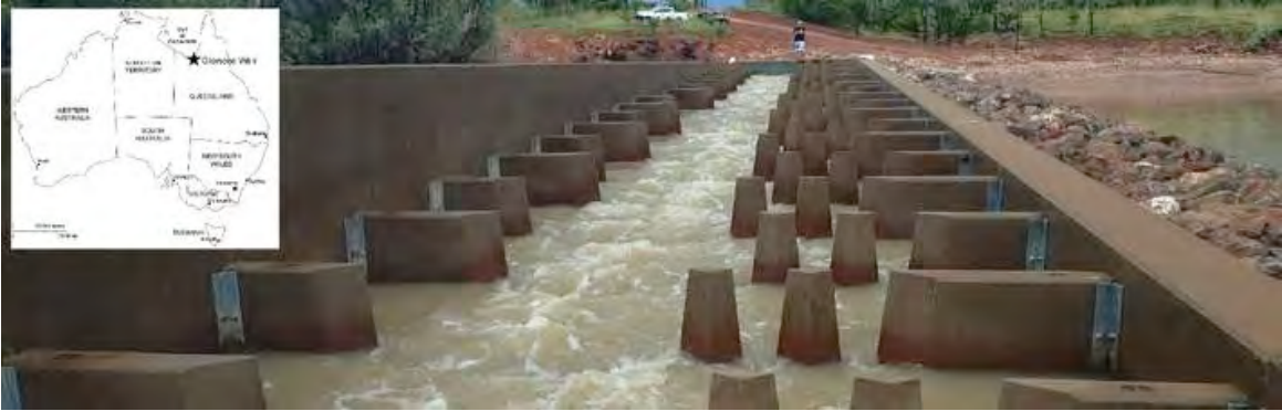
Above Glenore Weir Cone Fishway (high flow) located in the Southern Gulf of Carpentaria
