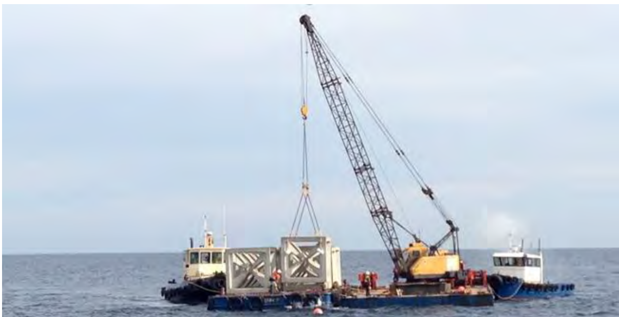
Figure 16: Crane and barge deployment of concrete artificial reef modules in Western Australia.
